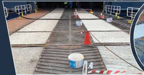
Main Ramp Lamination
